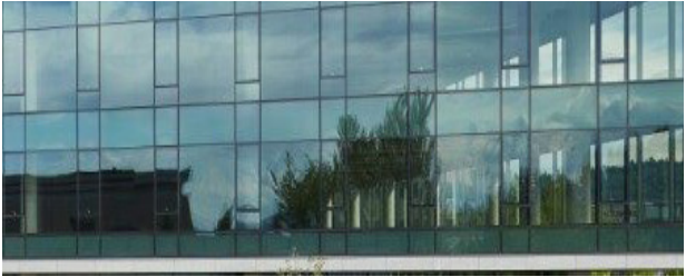
10 Typ. Curtain Wall Glass, Spandrel* Solarban 72 coating on Acuity glass Color: Light Gray Fritt on Surface #4 U Value: 0.29
