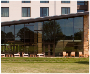
09.1 Curtain Wall Glass Solarban 72 coating on Acuity glass Color: Transparent with Low reflectivity U Value: 0.29
