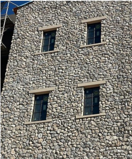
Cut Stone 1 ½" per plan Stucco Band at rock wall location
